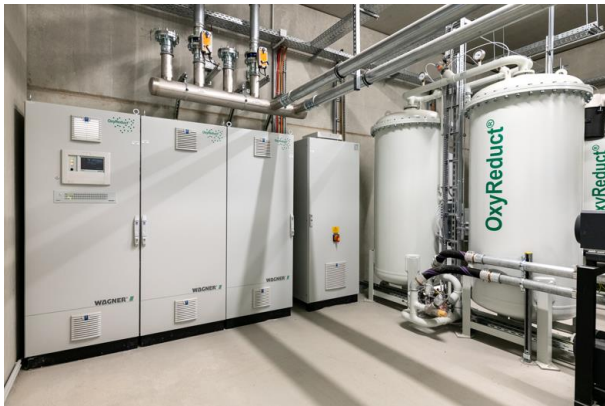
Caption: An OxyReduct® system for oxygen reduction protects automated compact storage systems against the development or spread of fire.
