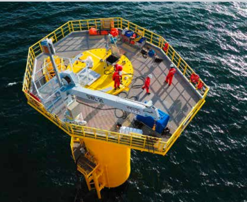
The platform is prepared for the installation of a wind turbine
