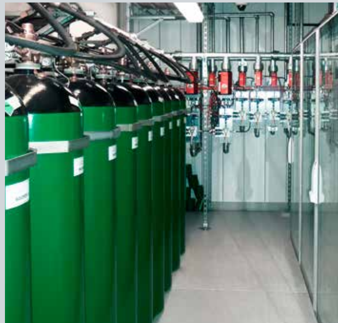
400 kg of nitrogen in cylinders for quick release in ten areas with areas between 10 and 100 m 2
